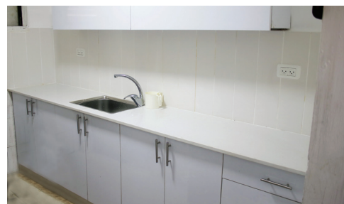
Kitchen after repairs
